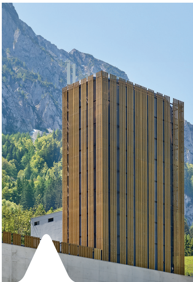
Bosruck Tunnel, Bosruck, Austria - Architect: Riepl Riepl Architekten - Copyright: Olaf Rohl - Product: Nordic Copper
